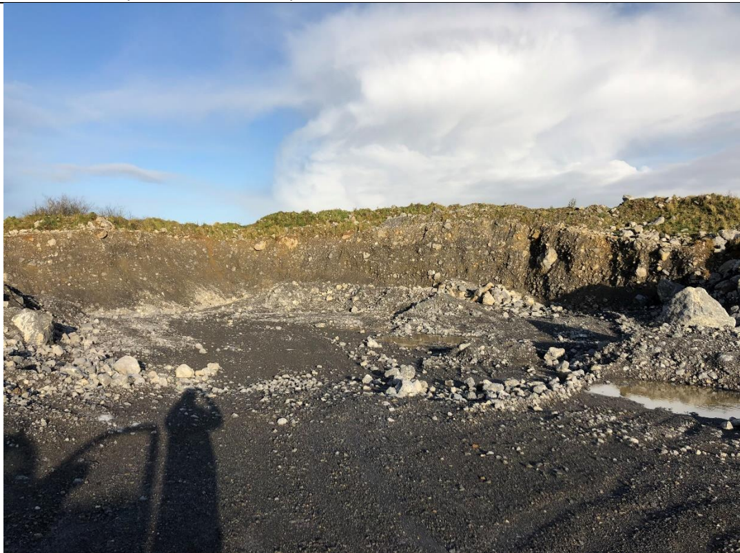
Site Photo 4: Overburden deposits at Cam Quarry showing large boulders close to ground level.
